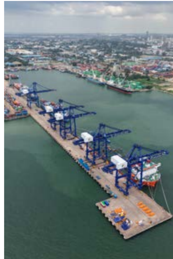
Batu Ampar Container Terminal
