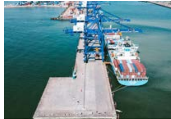
Batu Ampar Container Terminal
