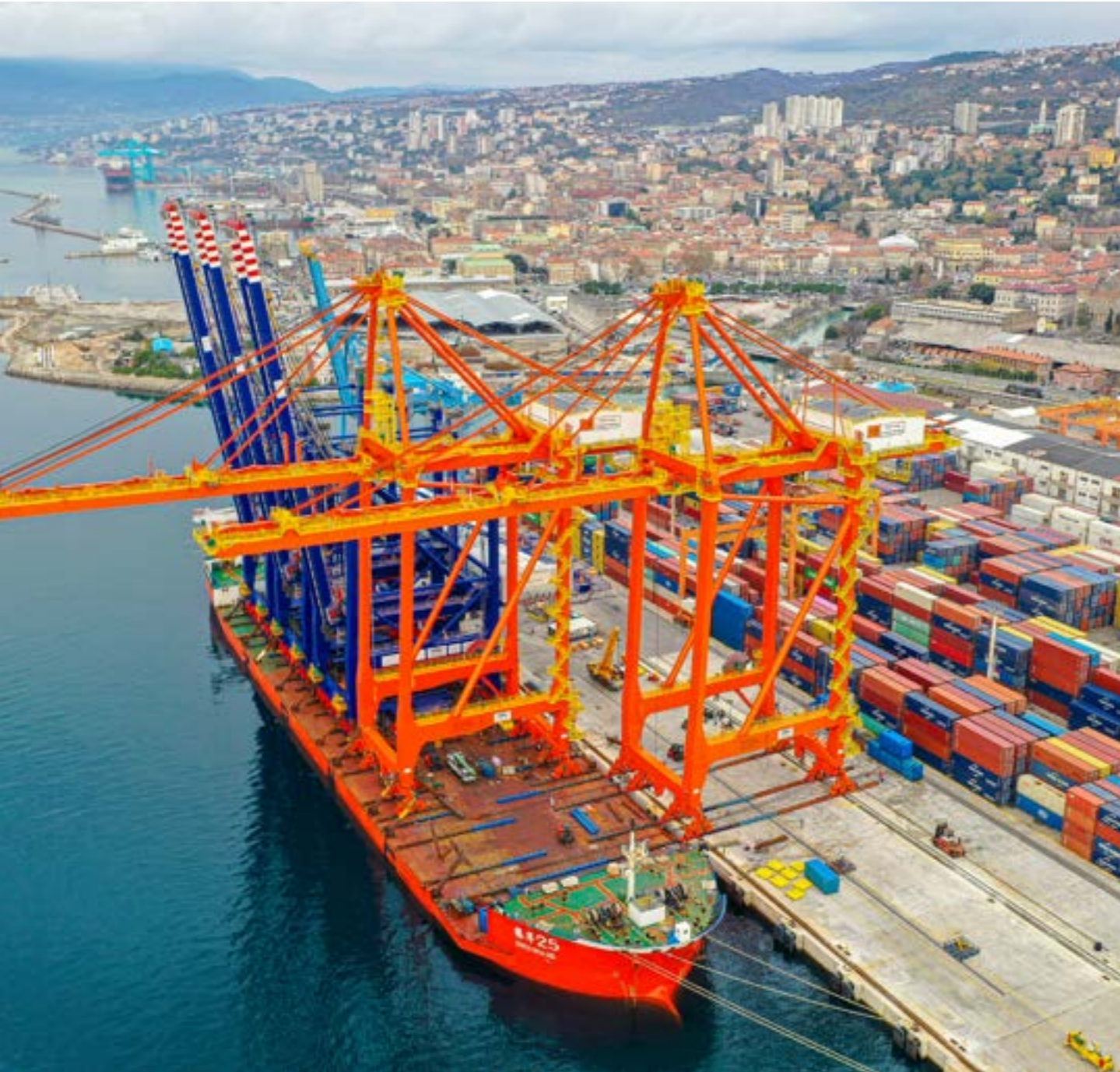
Adriatic Gate Container Terminal's new quay cranes enabled more efficient handling of larger vessels for faster turnaround times.
