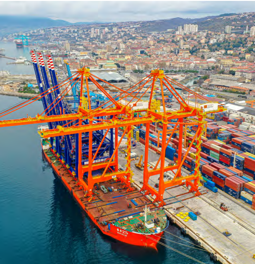
Adriatic Gate Container Terminal's new quay cranes enabled more efficient handling of larger vessels for faster turnaround times.
